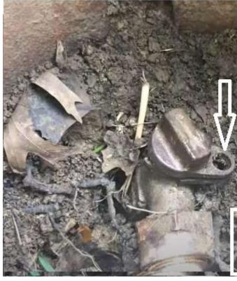
When the water valve is turned off, the holes on the valve will be lined up. This is for the lockout the water company will use when you don't pay your bill.
