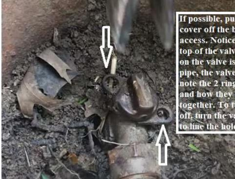
If possible, pull the entire cover off the base for better access. Notice the arrow on top of the valve. If the arrow on the valve is in line with the pipe, the valve is open. Also note the 2 rings on the valve and how they are not lined up together. To turn the valve off, turn the valve clockwise to line the holes up.
